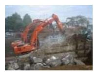
Demolition of redundant two lane solid concrete and steel constructed rail over bridge in Papakura. Sucessfully completed within a 24hour timeframe.
