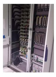
Fig3. Object control unit depicting the termination of fibres
